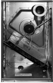
Heating Compartment Access
